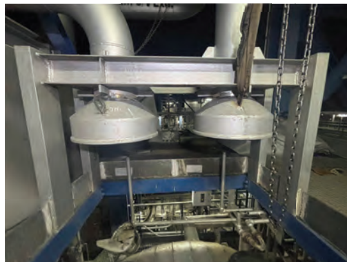
Install Safety Valve LP Drum
